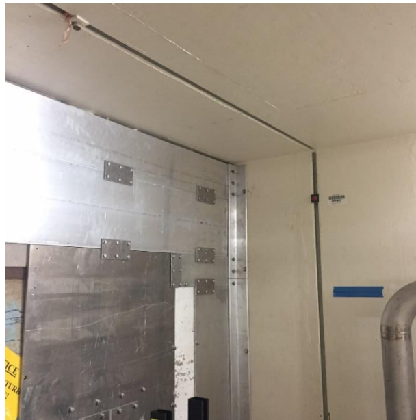
Example of Embedded Unistrut
